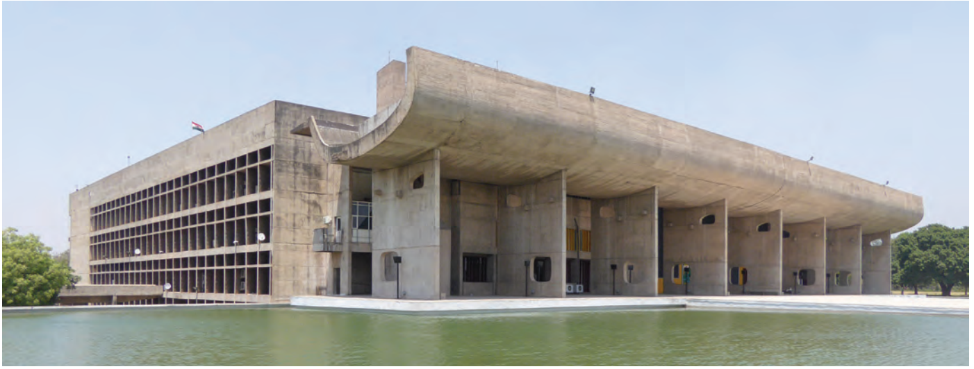
Fig. 2: Exposed concrete finish at the Legislative Assembly in Chandigarh, India, designed by Le Corbusier
