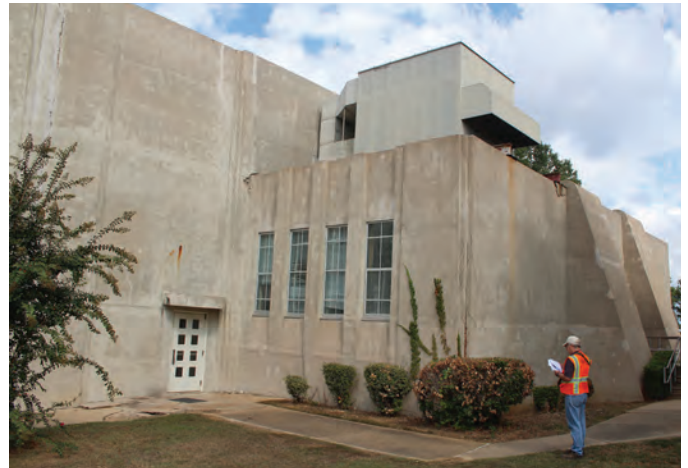
Fig. 7: Ongoing condition assessment of a historic concrete building facade
