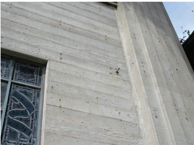
Fig. 6: Variations in formwork and finish at a historic concrete facade
