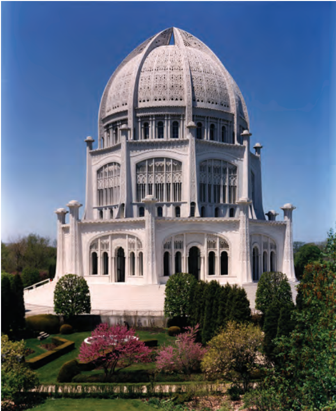
Fig. 1: Architectural precast concrete at the Bahai Temple in Chicago, Illinois, designed by Louis Bourgeois and John J. Earley
