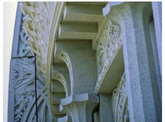
To repair the crown or clerestory cornice, technicians removed deteriorated architectural concrete and structural concrete. The finished repair matched the original
