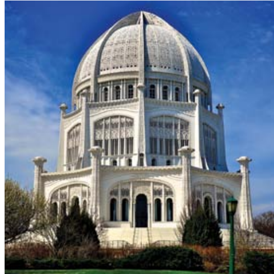
Twenty years after repairs, the Baha'i House of Worship's exquisite beauty continues to sparkle in the sunlight and dazzle hundreds of thousands of visitors each year
