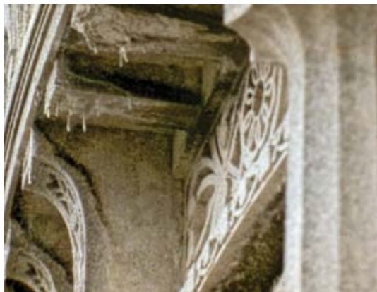
To repair the crown or clerestory cornice, technicians removed deteriorated architectural concrete and structural concrete. The finished repair matched the original
