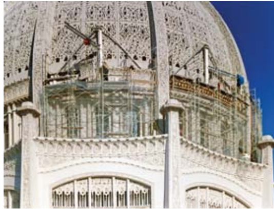
Special hoisting and access systems were designed for the concrete repairs
